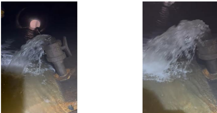
Figure 9: Effect of pulse application on sub-vertical drains inside a tunnel.
